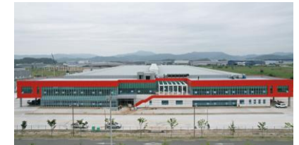
산업설비 (Industrial Facility)
