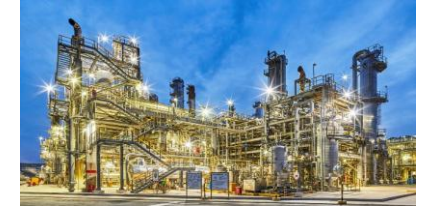
화공 (Chemical Plant)
