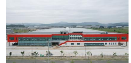
산업설비 (Industrial Facility)
