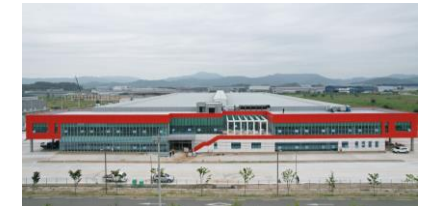
산업설비 (Industrial Facility)
