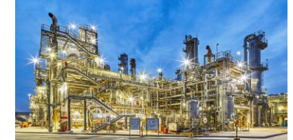
화공 (Chemical Plant)
