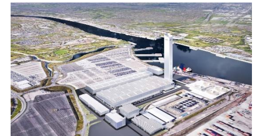
Bird's Eye View of New Submarine Cable Factory in England
