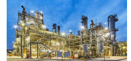
화공 (Chemical Plant)
