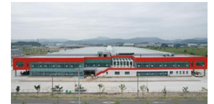
산업설비 (Industrial Facility)
