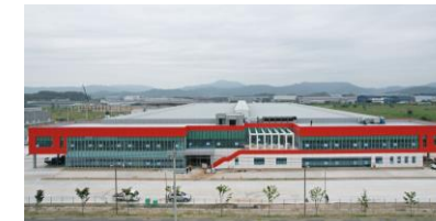
산업설비 (Industrial Facility)
