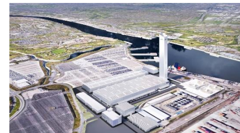
Bird's Eye View of New Submarine Cable Factory in England
