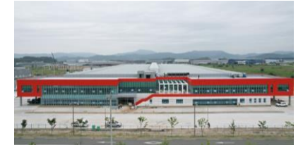
산업설비 (Industrial Facility)
