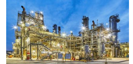
화공 (Chemical Plant)
