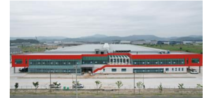
산업설비 (Industrial Facility)
