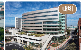
EmeryStation West Emeryville, CA
