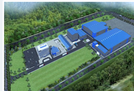
3rd Hydro Center (Under construction)
